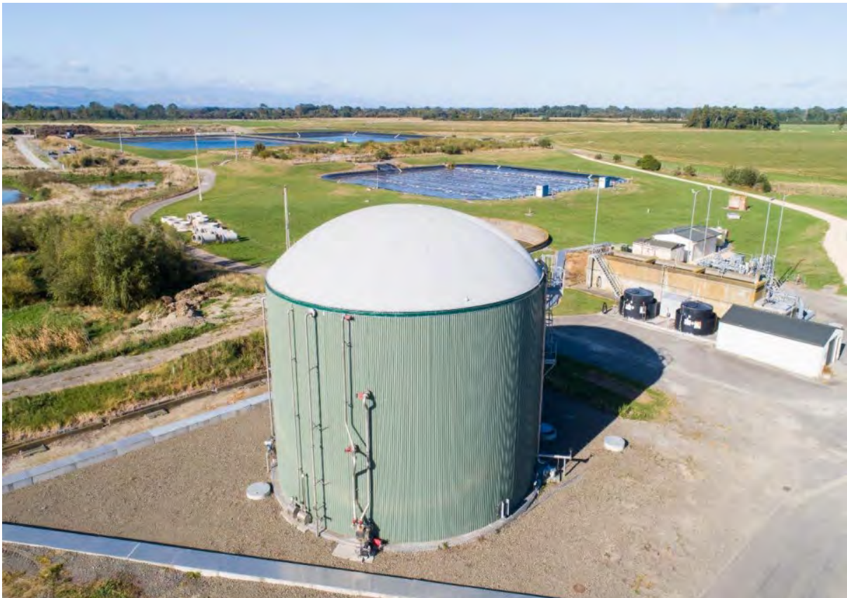
(Anaerobic digester at the Manawātū WWTP)
